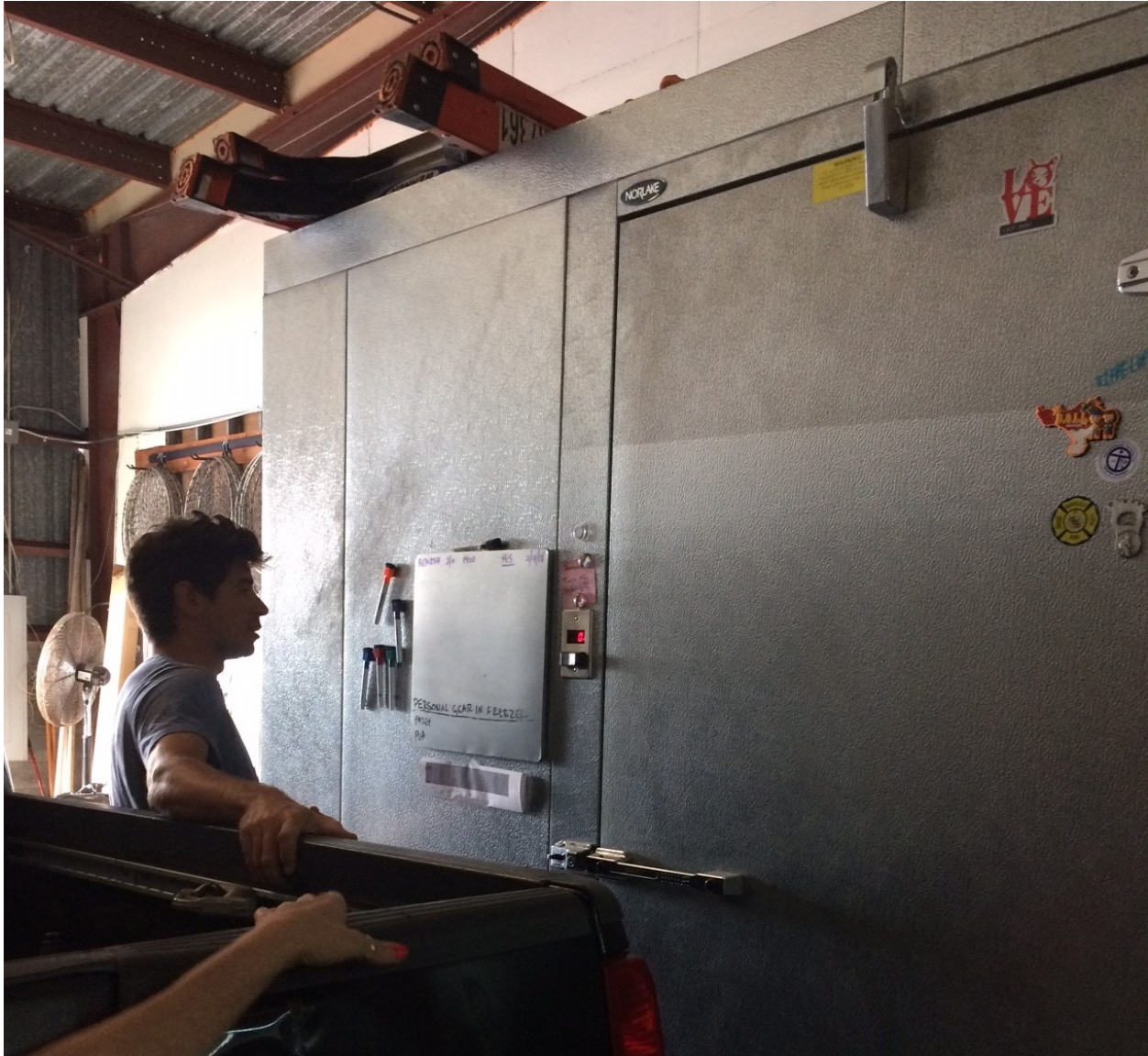
Figure 28 - Walk-in freezer at the PIROP gear shack in Honolulu.
