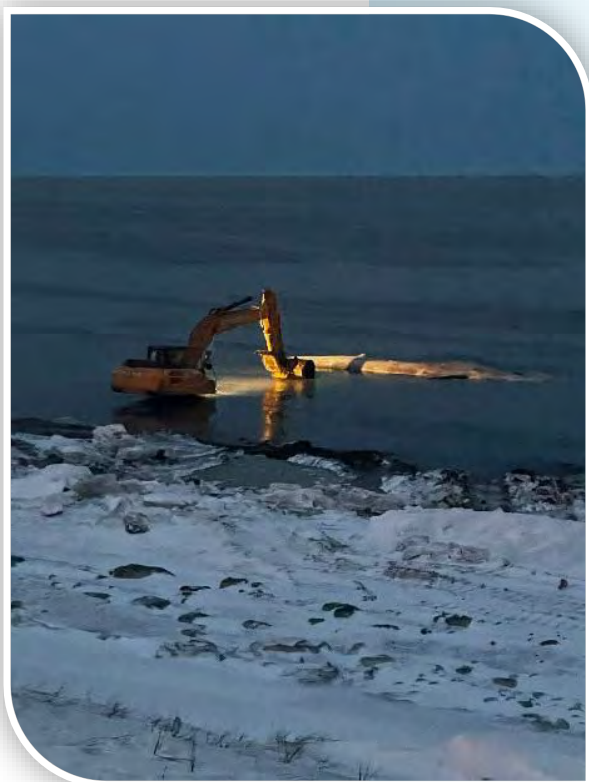
Heavy equipment used to push the whale off the beach.
