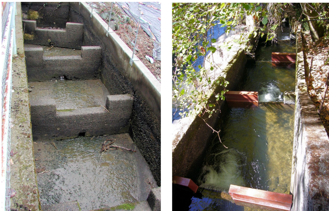
Figure 5-6. Examples of pool and weir ladders
