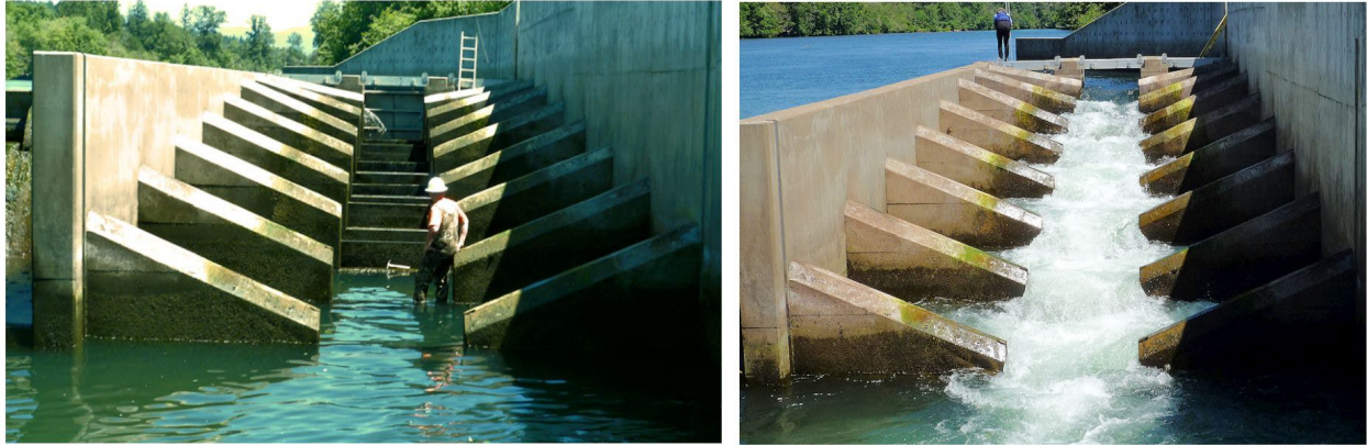
Figure 5-9. Pool and chute ladder dewatered (at left) and watered (at right)
