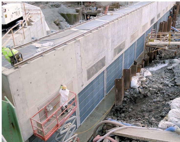
Figure 6-3. Picket barrier panels under construction at the Slide Creek tailrace barrier located on the North Umpqua River, Oregon
