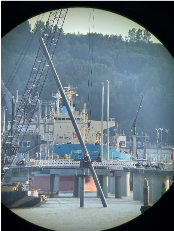
Photo 14. Preparing to install battered pile. View towards SFD from Ship Creek PSO station through Fujinon 25X150 MT-SX “big eyes”
