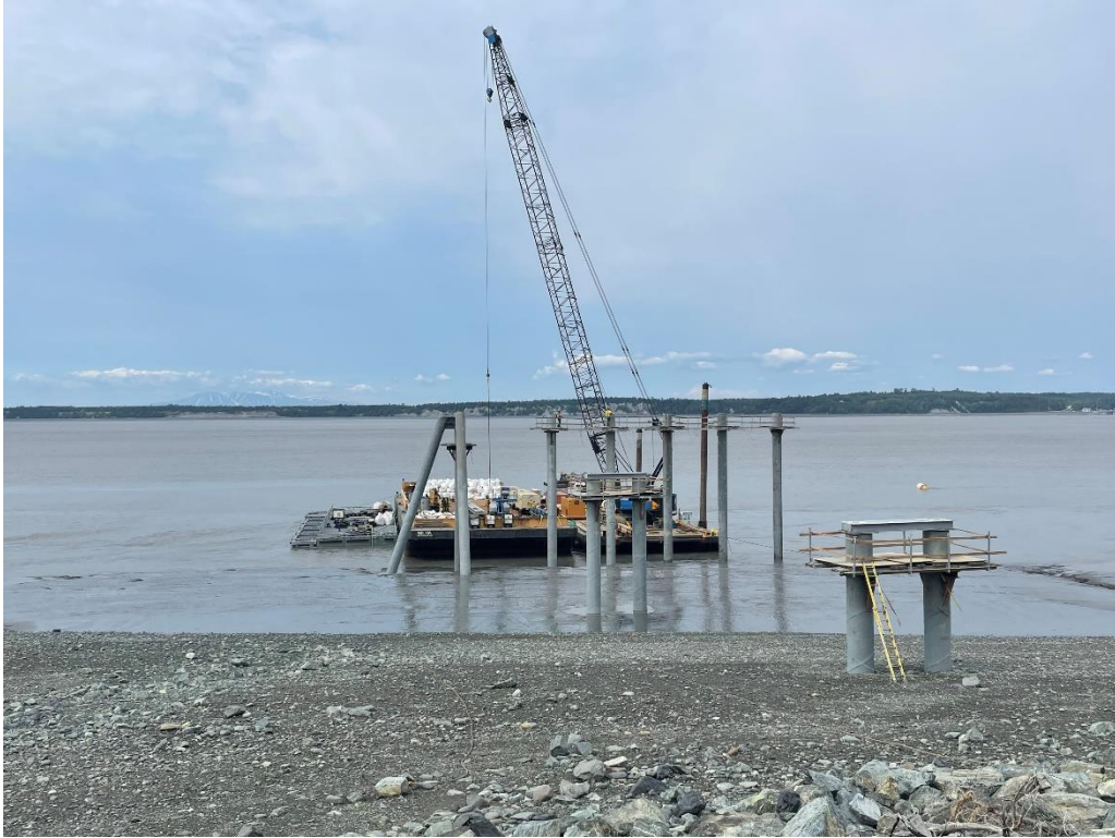
Photo 1. View of SFD construction from PCT PSO Station
