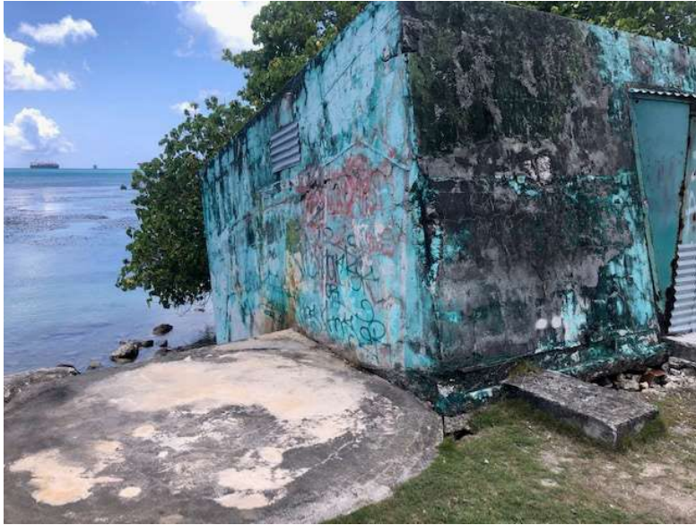
Figure E-5. Cement block structure and associated round cement pad to be demolished. Credit: NMFS, 2021.
