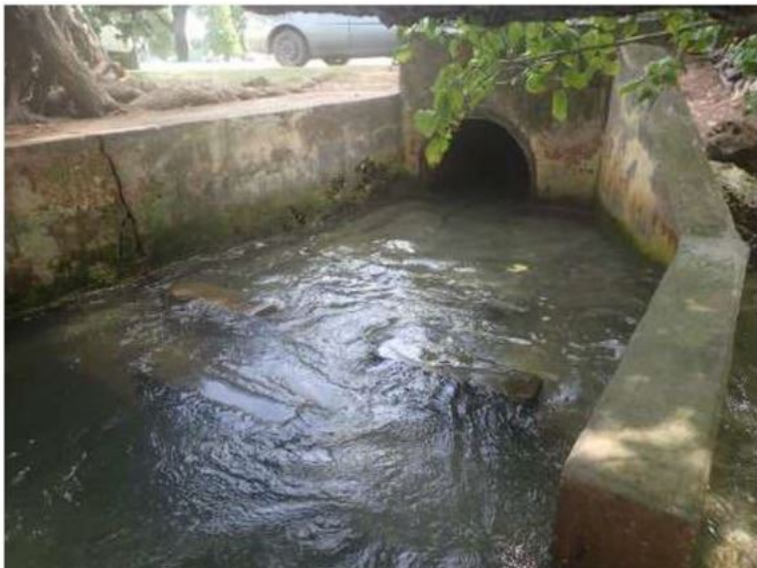
Figure 6. Storm drain adjacent to the revetment project site. Credit: DLNR 2021.
