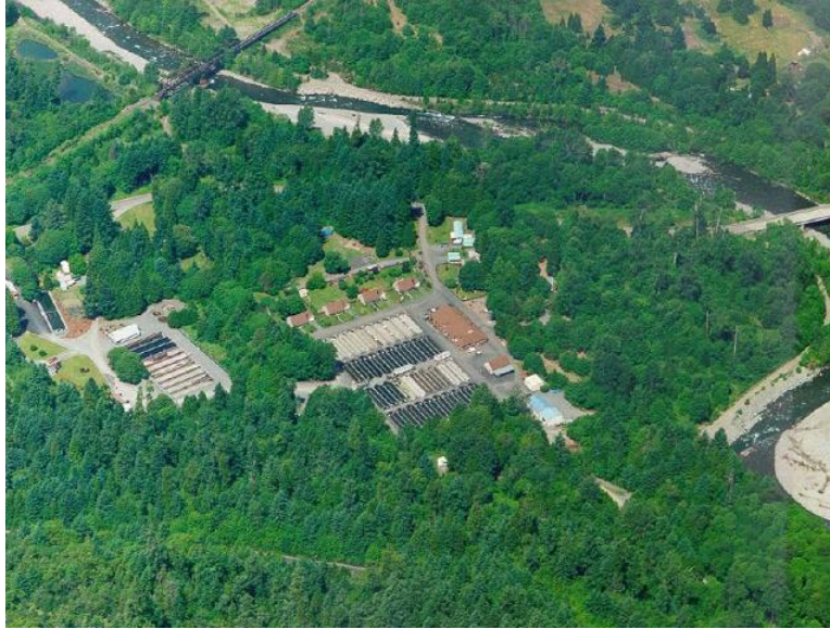
Figure 2-12 Willamette Hatchery Near Oakridge, Oregon.
